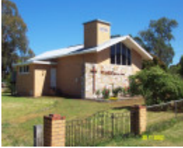
23656 St Mark s Anglican Church Cavendish 2077
