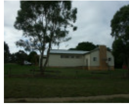
Corindhap Memorial Hall
