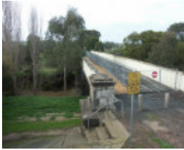
Iron Bridge over Leigh River
