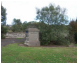
Iron Bridge over Leigh River
