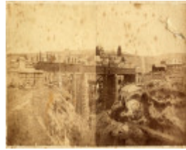
Shelford Bridge under construction, c.1874. Source: Dianne Hughes
