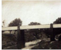
Iron Bridge, Shelford, c.1925. Source: Holmes collection c/o David Rowe.
