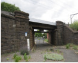
Bloomfield Road Rail Overbridge.JPG
