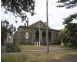
PORT FAIRY COURT HOUSE SOHE 2008
