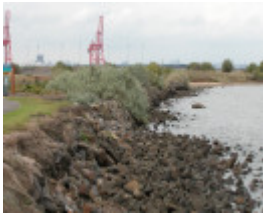
Newport Power Station Williamstown April 2003 Ash Pitt Walls 003
