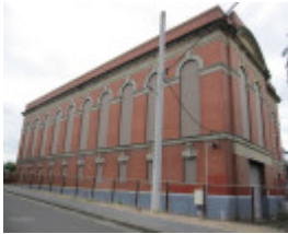
Newmarket Railway Substation.JPG
