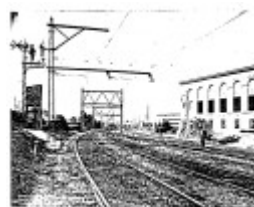
Newmarket railway yards and sub-station during electrification tests (SLV).
