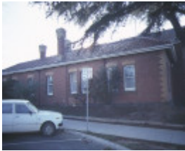
ararat court house side view jun1984
