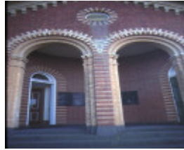
ararat court house entrance detail jun1984
