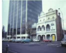
1 dalmeny house 21 queensberry street carlton street view jul1979
