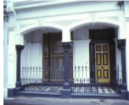
dalmeny house 21 queensberry street carlton front entrance jul1979
