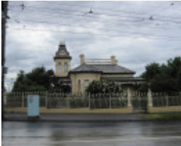
200 Pascoe Vale Road.JPG
