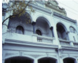
Cramond House 23 Queensberry Street Carlton balcony & arch detail Jul 1979
