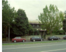
1 former presbyterian manse rathdowne street exterior sw apr1999
