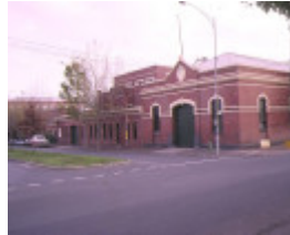
former cable tram engine house rathdowne street carlton north exterior of car shed corner view jun1995
