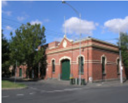
FORMER CABLE TRAM ENGINE HOUSE SOHE 2008
