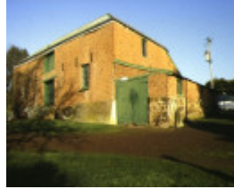
1 red brick barn late 1840s muntham casterton side view
