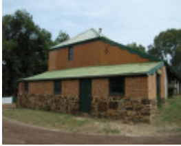
RED BRICK BARN SOHE 2008
