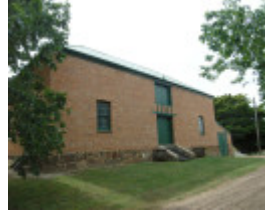
RED BRICK BARN SOHE 2008
