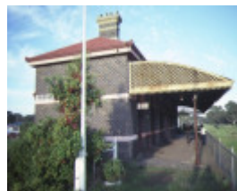
casterton railway station side view jun1984
