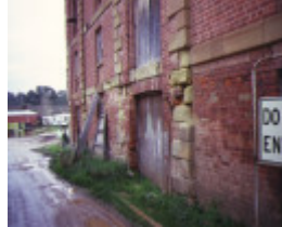
flour mill barker street castlemaine brickwork detail
