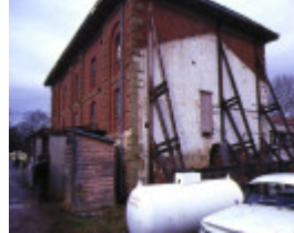
1 flour mill barker street castlemaine front view
