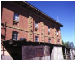
flour mill barker street castlemaine rear view
