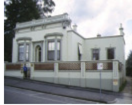
1 medical rooms mostyn street castlemaine front view
