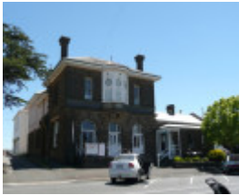
FORMER ARARAT SUB-TREASURY AND POST OFFICE SOHE 2008
