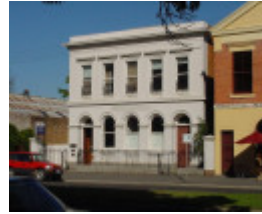
H00131 1 former bank of nsw castlemaine front elevation 2002
