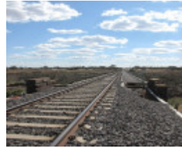
2504_Melton Railway Viaduct_7 November 2009_HV_072_lo res.jpg
