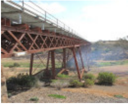
2504_Melton Railway Viaduct_7 November 2009_HV_069_lo res.jpg
