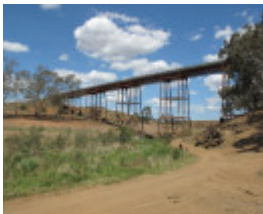
2504_Melton Railway Viaduct_7 November 2009_HV_007_lo res.jpg
