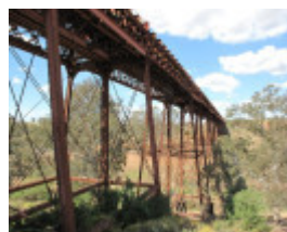
2504_Melton Railway Viaduct_7 November 2009_HV_030_lo res.jpg
