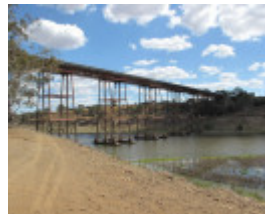
2504_Melton Railway Viaduct_7 November 2009_HV_009_lo res.jpg
