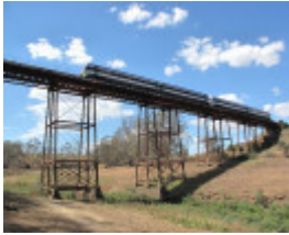
2504_Melton Railway Viaduct_7 November 2009_HV_041_lo res.jpg
