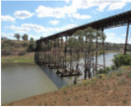
2504_Melton Railway Viaduct_7 November 2009_HV_032_lo res.jpg
