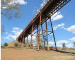
2504_Melton Railway Viaduct_7 November 2009_HV_058_lo res.jpg
