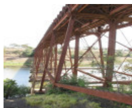
2504_Melton Railway Viaduct_7 November 2009_HV_026_lo res.jpg
