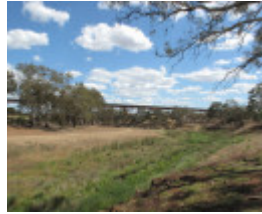
2504_Melton Railway Viaduct_7 November 2009_HV_005_lo res.jpg
