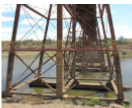
2504_Melton Railway Viaduct_7 November 2009_HV_019_lo res.jpg
