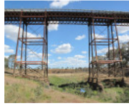
2504_Melton Railway Viaduct_7 November 2009_HV_056_lo res.jpg
