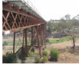
2504_Melton Railway Viaduct_7 November 2009_HV_070_lo res.jpg
