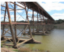
2504_Melton Railway Viaduct_7 November 2009_HV_013_lo res.jpg
