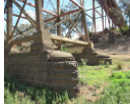
2504_Melton Railway Viaduct_7 November 2009_HV_055_lo res.jpg
