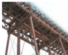
2504_Melton Railway Viaduct_7 November 2009_HV_016_lo res.jpg
