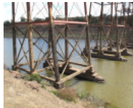
2504_Melton Railway Viaduct_7 November 2009_HV_012_lo res.jpg
