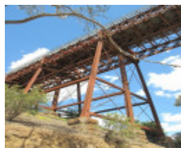
2504_Melton Railway Viaduct_7 November 2009_HV_017_lo res.jpg
