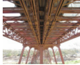
2504_Melton Railway Viaduct_7 November 2009_HV_068_lo res.jpg
