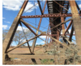
2504_Melton Railway Viaduct_7 November 2009_HV_048_lo res.jpg
