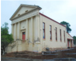
FORMER EAGLEHAWK EAST METHODIST CHURCH SOHE 2008
