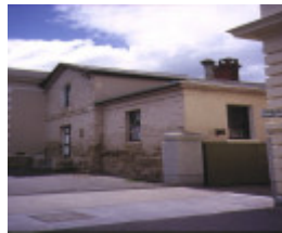
former telegraph office and faulder watson hall barker street castlemaine side view telegraph office
