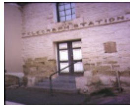
former telegraph office & faulder watson hall barker street castlemaine front view telegraph office
