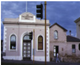
former telegraph office & faulder watson hall barker street castlemaine front view faulder watson hall
