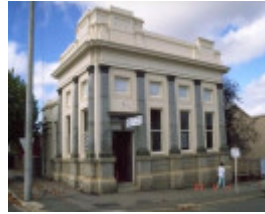
h00580 former state savings bank h0580
