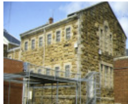
former hm prison challis street castlemaine rear view of cell block
