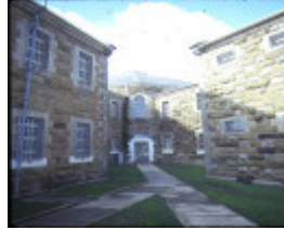
1 former hm prison challis street castlemaine cell block entrance aug1984
