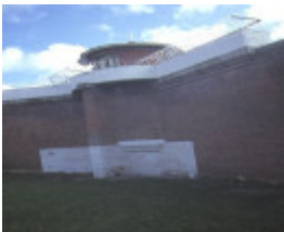
former hm prison challis street castlemaine watch tower & walls aug1984
