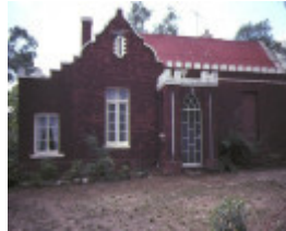
residence farnsworth street castlemaine side view may1984
