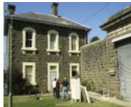
mental hospital ararat front gate & gatehouse
