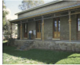
1 former castlemaine court house goldsmith crescent castlemaine front view
