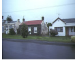
1 cottage 64 campbell street port fairy front view
