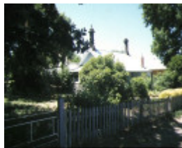
chatsworth lodge johnstone street castlemaine view front street
