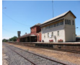
Wangaratta RWS Signal Box & Station Building February 2002
