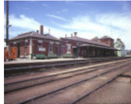
1 wangaratta railway station complex norton street wangaratta trackside view dec1984
