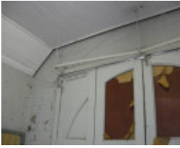
Timber-boarded ceiling junction with south and west walls inside the former fire engine room
