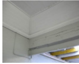
Steel lintel supporting a remnant of the 1896 building's east wall in the north-east corner of the former fire engine room
