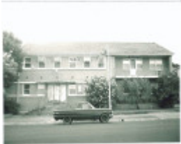
26491 New Police Station
