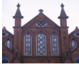
congregational church lyttleton street castlemaine detail front congregational church
