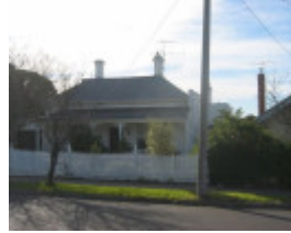
192 Wood Street, Preston
