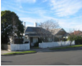
192 Wood Street, Preston
