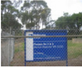
MMBW Preston Reservoir Complex, High Street, Reservoir
