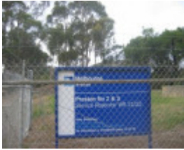
MMBW Preston Reservoir Complex, High Street, Reservoir
