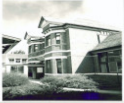
26621 Hamilton Base Hospital
