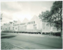
26678 Permewan Wright Sheds
