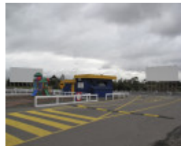
Coburg Drive In_8 May 2009_mz_Projection Building and Screens 2 and 3
