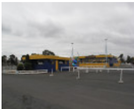
Coburg Drive In_8 May 2009_mz_Diner and Projection Building
