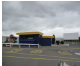
Coburg Drive In_8 May 2009_mz_Projection Building
