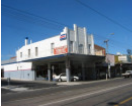
Drive in Service Station, 802 High Street
