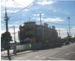
Junction Hotel, 2 - 4 High Street, Preston
