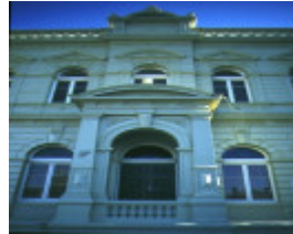
1 former school of mines lyttleton street castlemaine entrance
