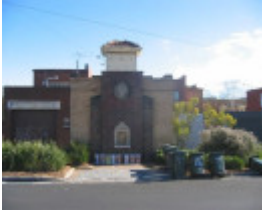
Electricity Substation, Pender Street, Thornbury
