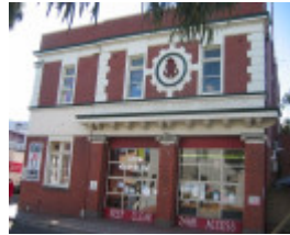
378 High St - Metropolitan Fire Brigade
