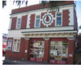
378 High St - Metropolitan Fire Brigade
