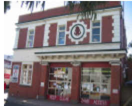
378 High St - Metropolitan Fire Brigade
