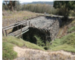
H2167 Lady Northcote Camp Sewerage System
