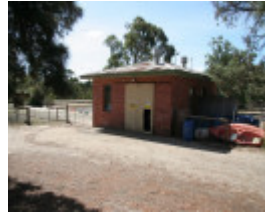
H2167 Lady Northcote Camp Maintenance Shed
