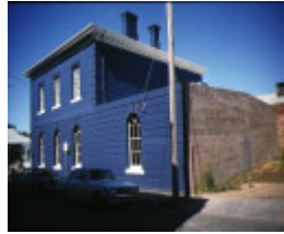
former bank of australasia mostyn street castlemaine side view
