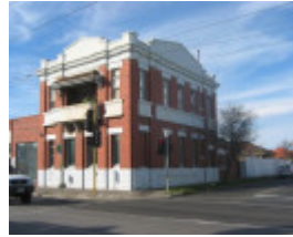
State Saving Bank (Former), 600-606 Plenty Road, Image 2
