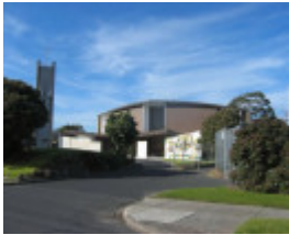
Holy Name Catholic Primary School & Church, 2-26 Robb Street, Preston
