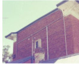
ferndale manor castlemaine rear elevation
