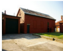
H2170 St Vincent de Paul Boys Orphanage c 1866 timber classroom
