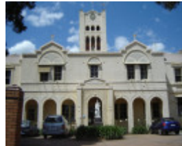
st vincent's boys orphanage sth Melbourne front entrance
