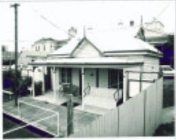
27233 Bowling Club Rooms
